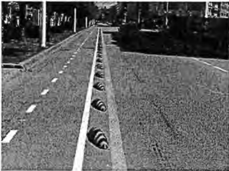
Armadillo 5" tall – can be rolled over in larger vehicles
