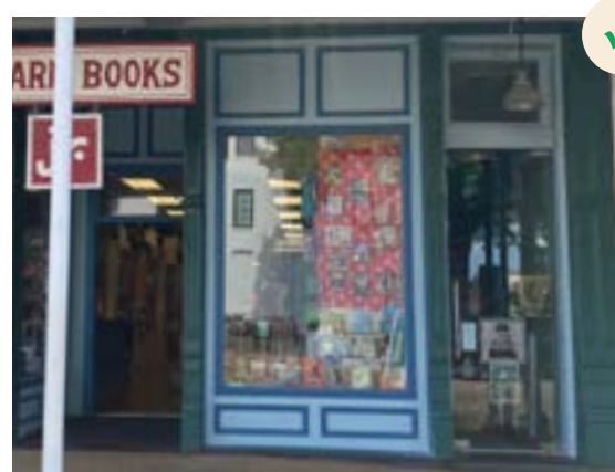
This new door does not copy what may have been the original door style (possibly a wooden, single-lite door), but the new door is also secondary to the historic entrance and does not detract from the rhythm of the storefront.
