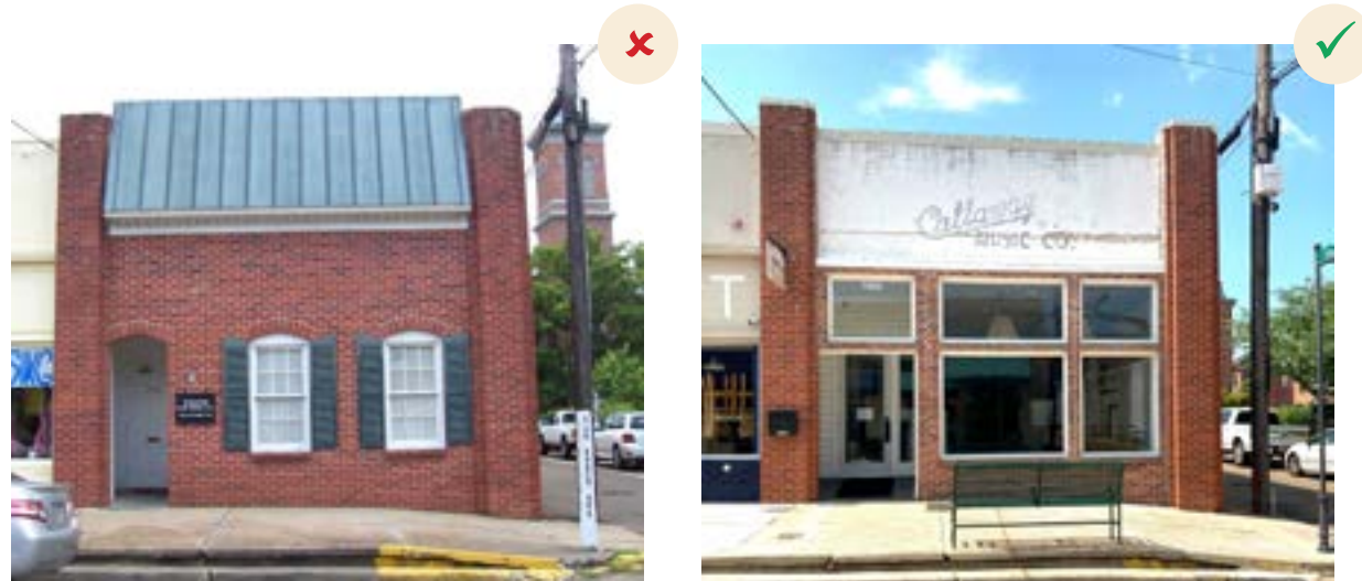
The new Storefront openings echo possible size and placement of original openings and continue the rhythm of the windows on the street.
