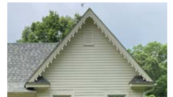
New construction in 2019 at 1224 Johnson Avenue
