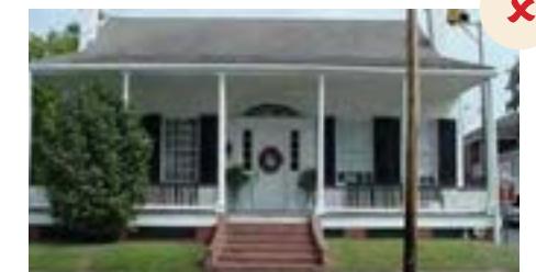
Original wood entry steps replaced by brick steps divert attention from the original detailing of the house.
