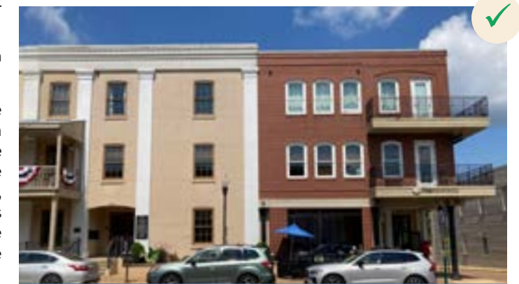
A new addition to the Historic Thompson House is compatible to the original structure in scale, rhythm and height while differentiating the addition with the use of materials and simplified ornament and detail.
