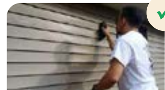
Hand wash siding to prevent water infiltration beyond the siding.
