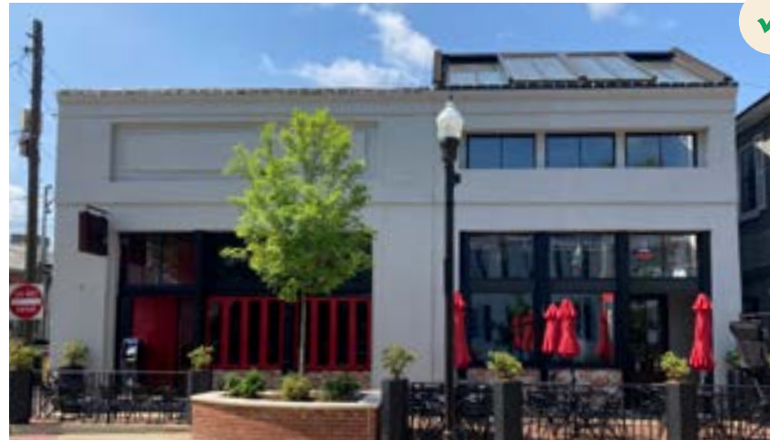
Funky's is an example of appropriate scale, rhythm, height and detail for new infill design and construction.
