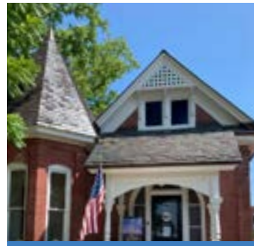
The shape and slate tiles are significant characteristics of this roof.
