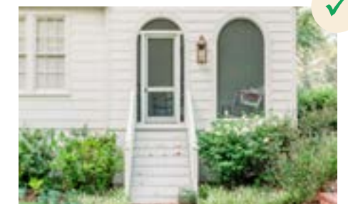
Original wood entry steps replaced by new wood entry steps.
