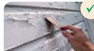
Scrape paint by hand for regularly needed maintenance
