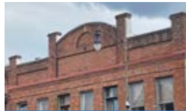
Picture of a pretty brick parapet.
