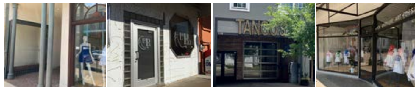
The images above are examples of how innovations in glass technology have impacted storefronts in Oxford. Mirrored glass, glass block, aluminum roll-up doors, and large expanses of plate glass.
