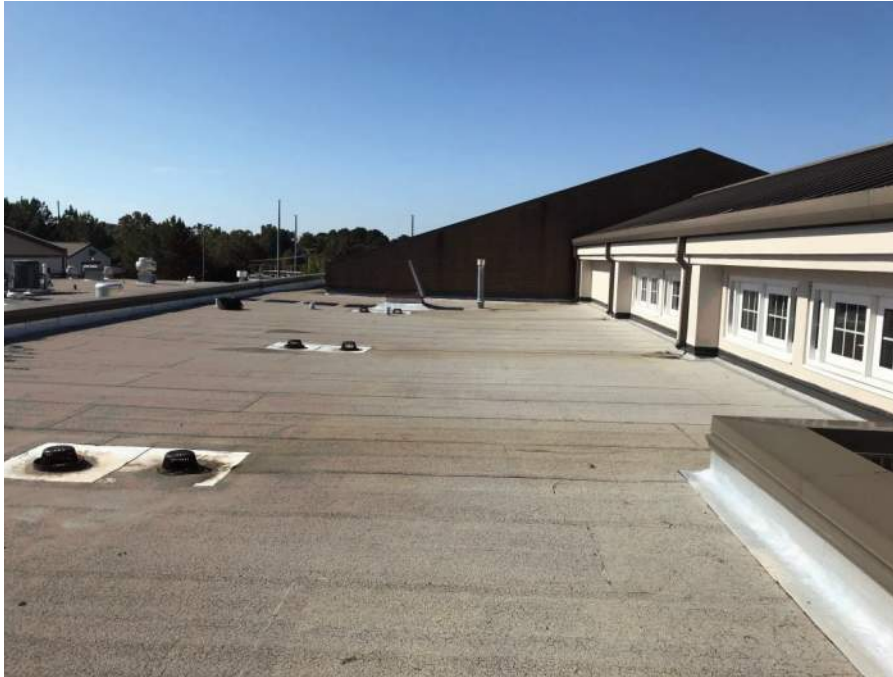
Item #1D: Roof D – Overall view
