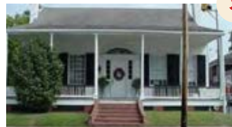
Original wood entry steps replaced by brick steps divert attention from the original detailing of the house.
