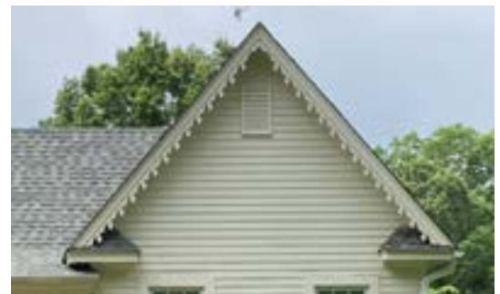
New construction in 2019 at 1224 Johnson Avenue
