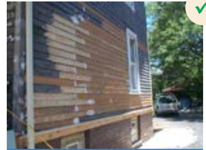
Replace only areas of wood that are deteriorated.
