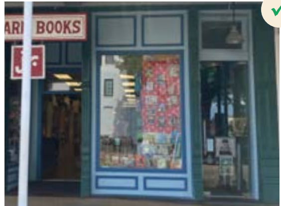
This new door does not copy what may have been the original door style (possibly a wooden, single-lite door), but the new door is also secondary to the historic entrance and does not detract from the rhythm of the storefront.
