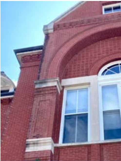
Brick can be decorative as well as functional with some buildings featuring brick cornices, recessed brick panels, brick arches defining windows and doors, and patterned brickwork.
