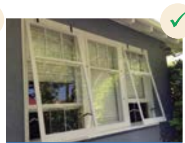
The rail on the storm window aligns with the meeting rail of the original window. These storm windows are easily removable with minimal damage to the original casing.
