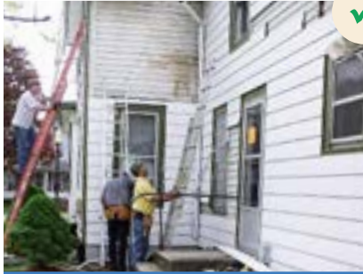
Remove vinyl siding to uncover wood original wood.
