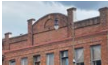
Picture of a pretty brick parapet.
