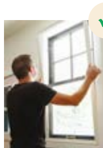
A compression fit interior storm window does not change the appearance of the window from the exterior and does not damage the existing window frame.
