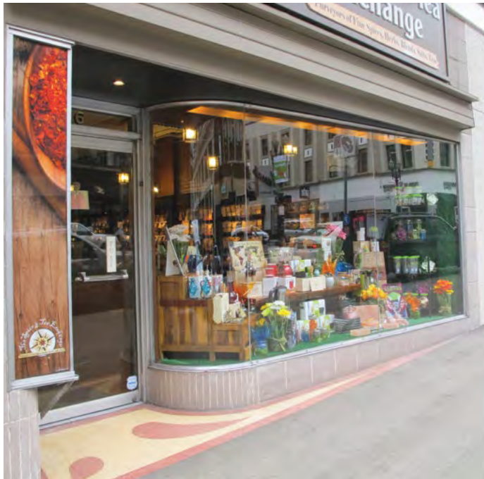
[27] This original c. 1940s storefront, with its character-defining angled and curved glass display window and recessed entrance with a decorative terrazzo paving, is in good condition and should be retained in a rehabilitation project.
