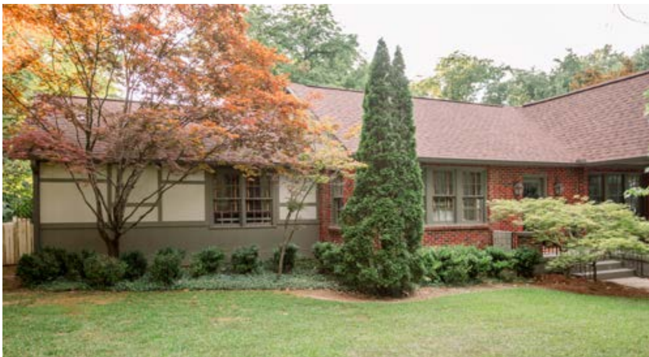
1428 S. 10th St. c. 1925 with a side and rear addition c. 1960
