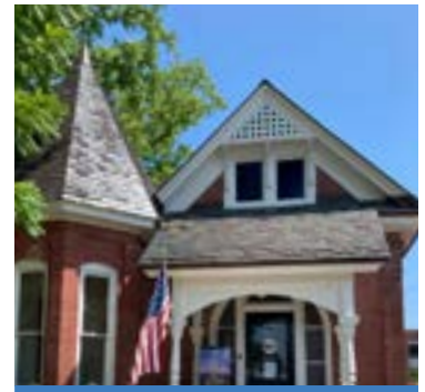
The shape and slate tiles are significant characteristics of this roof.
