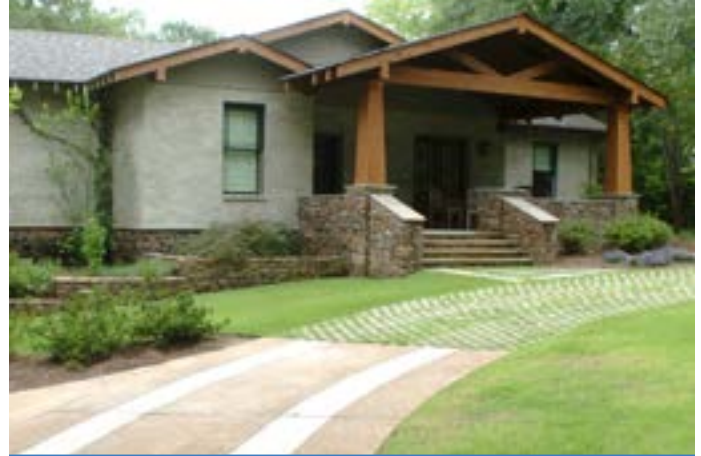
Pervious pavers were used in this circle drive to minimize the appearance of the drive in the front of the house. Exposed aggregate concrete and concrete were also used.
