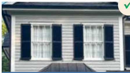
Appropriate shutters are compatible with the architectural style of the home and precisely cover the window when closed.
