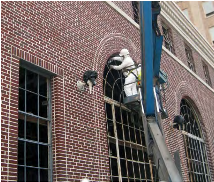
[57] Workers wear protective clothing while removing lead paint from metal features.
