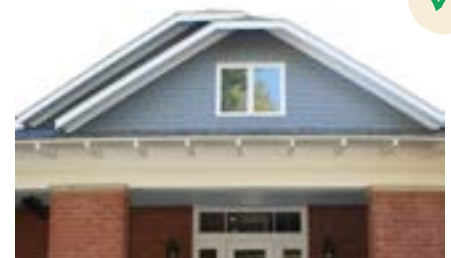
The "dogear" detail of this roof is a character-defining feature of the house. Shingles and the dogear detail are appropriate for the Craftsman style.
