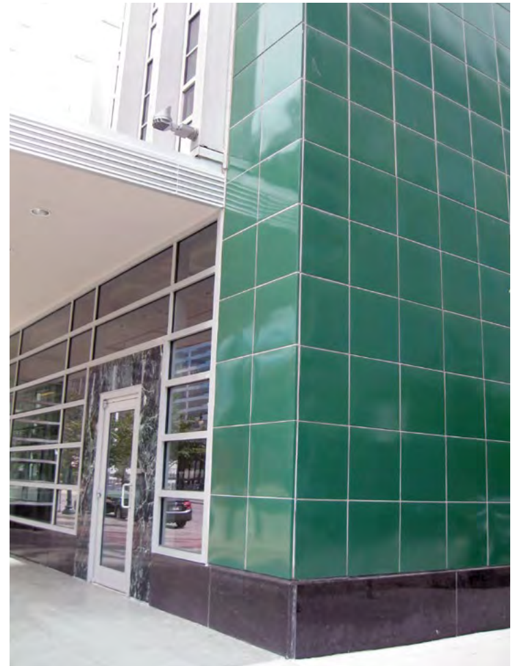
[15] New enameled-metal panels were replicated to replace the original panels, which were too deteriorated to repair, when the storefront of this early 1950s building was recreated.
