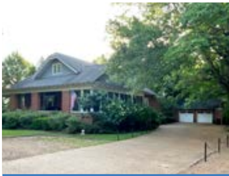
A new garage located at the rear of the site is subservient in scale to the historic residence at 650 N. Lamar Blvd.
