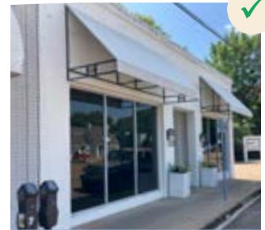
Awnings should have a 30-50 degree angle. Use shed awnings with open ends so the architectural detail behind the awning is still visible.
