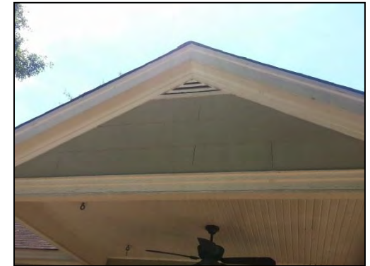
Pitch of house roof
