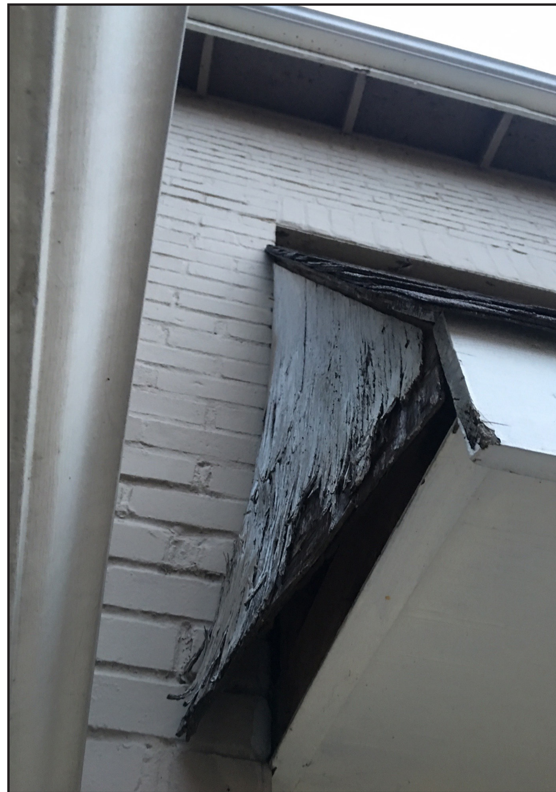
DETERIORATED AWNING
